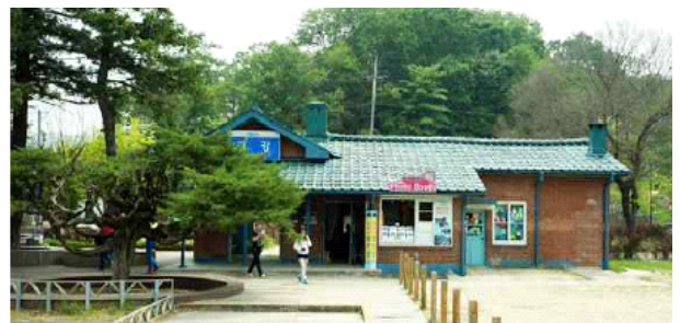
Figure 2. Gyeonggang Station (Current)
